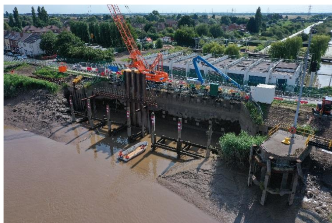
New outfall works
