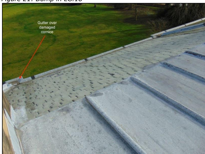
Figure 23: Gutter over damaged cornice
