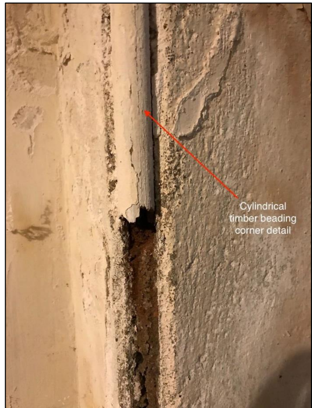
Figure 20: Corners of plaster finished walls to the corridor are formed with a cylindrical timber beading detail. Such details will be replicated as part of the proposed works
