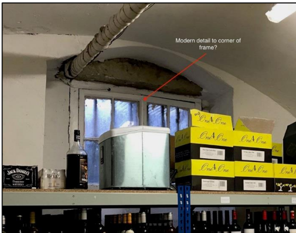
Figure 19: Probable 20 th century window to current wine store at LG.15. It is not shown on the 1974 floor plans
