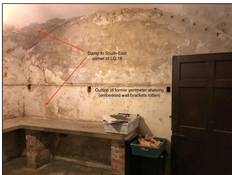
Figure 21: Damp in LG.18
