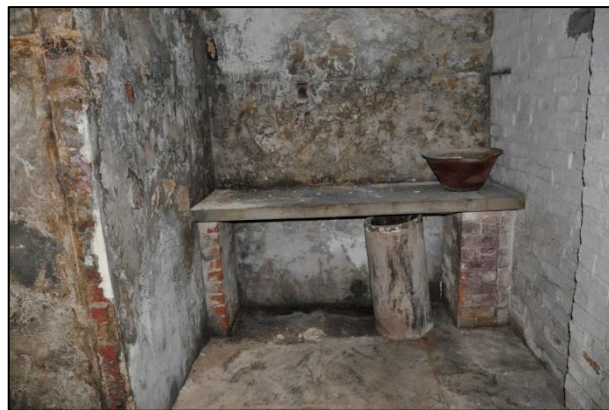
Figure 10: Part of further historical shelving in former larder or cold store adjacent to the wine cellar with stone slab supported on brick pier
