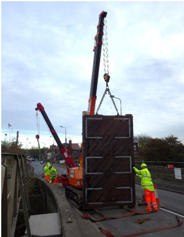
Above and right: The new tidal doors being installed at South Ferriby
