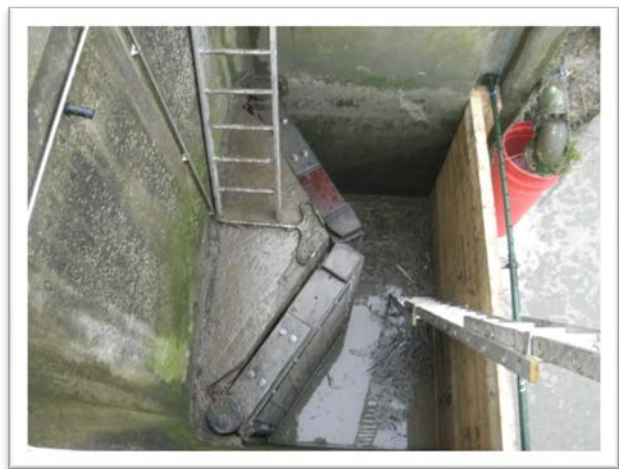
New tidal doors installed
