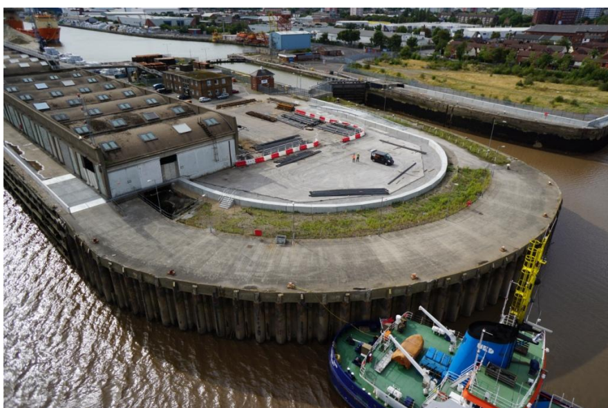
An aerial view of some of the new flood walls at Albert Dock
